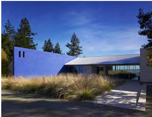
The blue wall's surface is stucco with gravel in the mix to create a rough-textured surface. The wall was painted with coats of blue paint. The dramatic hue was custom-designed by Fernandez, who closely guards the secret of his special color palette.
