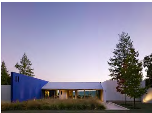
The house was designed to be almost transparent, with natural light and fresh air. An elongated blue stucco wall punctuates the low-slung residence. A concrete path leads to a pivoting glass front door. To the left of the wall is the garage. Construction: Grassi and Associates, Napa.
